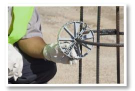
The table below illustrates the recommended number of Quick-Lock<sup>®</sup> Pier Wheels to be used on a per shaft basis. The actual number can vary subject to the number of vertical bars of the reinforcing steel cage. The structural engineer is the governing authority. When in doubt, please check with the structural engineer.
