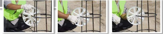
The table below illustrates the recommended number of Quick-Lock HD<sup>®</sup> wheels to be used on a per shaft basis. The actual number can vary subject to the number of vertical bars of the reinforcing steel cage. The structural engineer is the governing authority. When in doubt, please check with the structural engineer.
