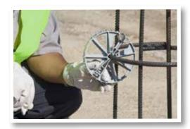
The table below illustrates the recommended number of Quick-Lock™ Pier Wheels to be used on a per shaft basis.
